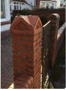
Brick pillars, decorative coping.
