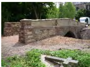
Prichard Bridge repair and refurbishment in 2012/13.
