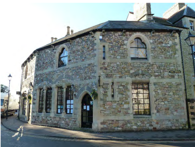
Polychromatic semi-coursed stone with Bath stone ashlar dressings: High Street.
