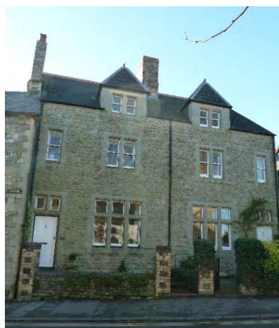
Thinly coursed greenstone: Cathedral Green.
