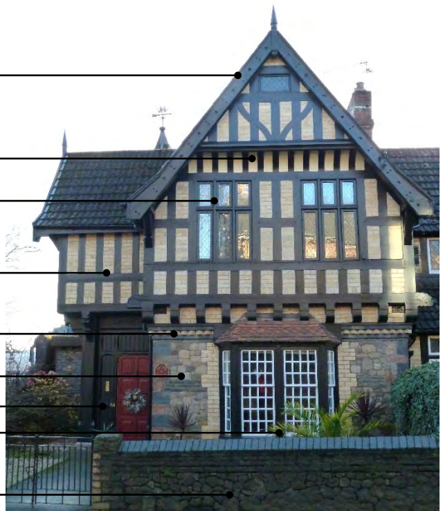
End 19 th century, likely architect George Halliday. Style of half-timbered Tudor domestic architecture.
