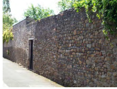
Historic rubble stone wall.
